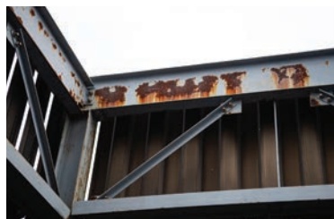
Clockwise from left: A water heater original to the building (1970); a rusted steam line connection; and rust on a steel structure on the building roof.
