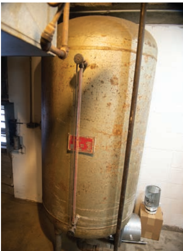
Clockwise from left: A water heater original to the building (1970); a rusted steam line connection; and rust on a steel structure on the building roof.
