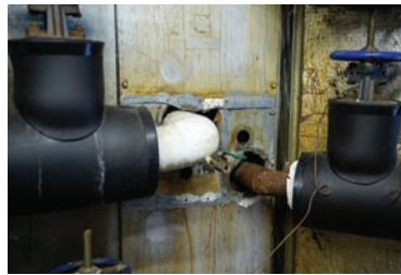
Clockwise from top: Exposed insulation on an air handling duct; rusting water on pipes; and a rusted steam conduit, all in the Nursing Education building.
