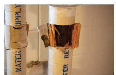
Clockwise from top: Exposed insulation on an air handling duct; rusting water on pipes; and a rusted steam conduit, all in the Nursing Education building.
